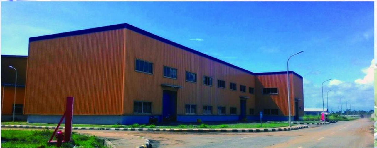
Auxiliary PLTU Nagan Raya Project - Building Area Workshop - Suak Puntong Village Location Nagan Raya District, Nanggroe Aceh Darussalam
