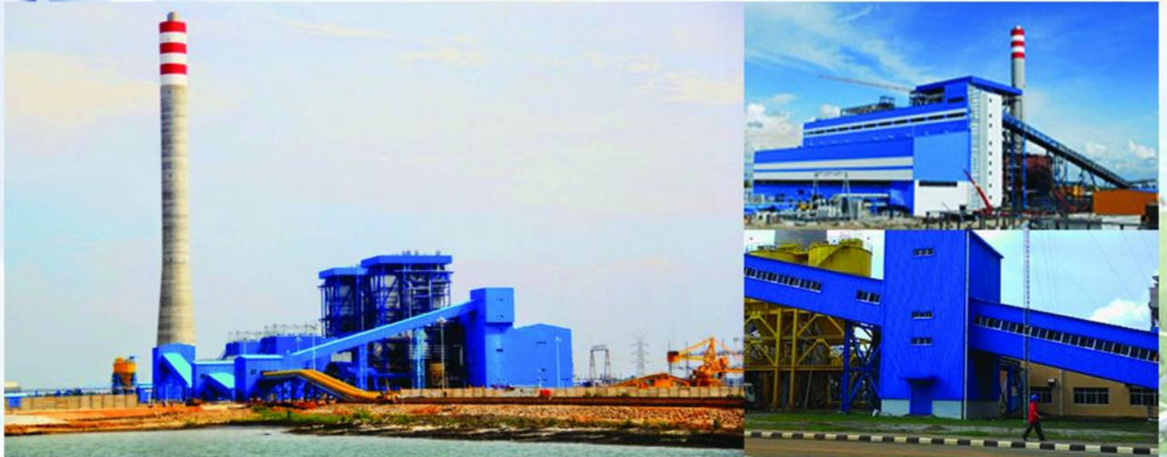
PLTU Nagan Raya Project - Location of Suak Puntong Village, Nagan Raya District, Nanggroe Aceh Darussalam
