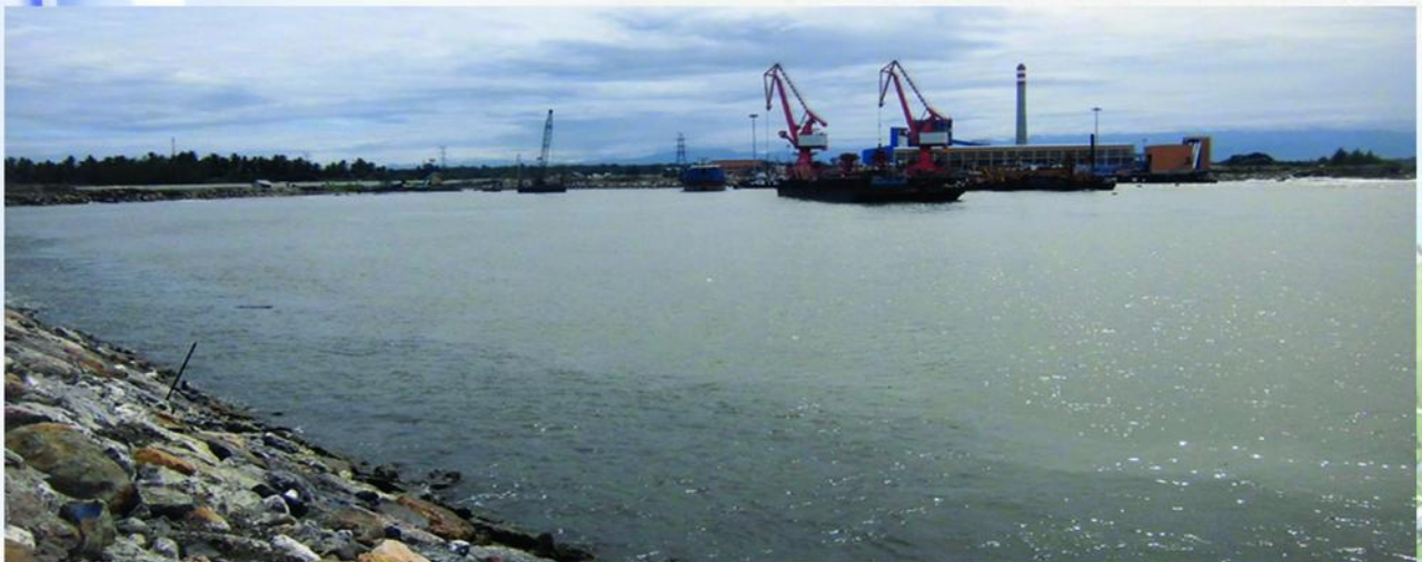
Taking Over Jetty PLTU Nagan Raya Project - Location Suak Puntong Village Nagan Raya District, Nanggroe Aceh Darussalam
