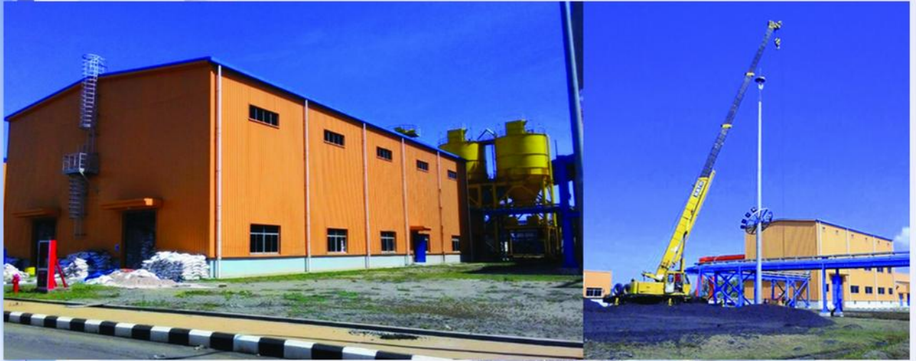
Auxiliary PLTU Nagan Raya Project - Limestone Building - Suak Puntong Village Location Nagan Raya District, Nanggroe Aceh Darussalam
